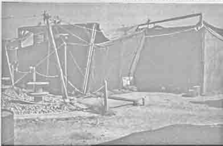
Above: The operating tent did not inspire confidence at first, but it did stay up. Plans were afoot to replace it with an aluminium hut but the casualties from the attack on Salalah were treated under canvas.
